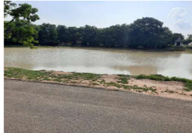
Hydrological problem in Melaselvanur pond: water loss is through evaporating, need recharge shafts.
