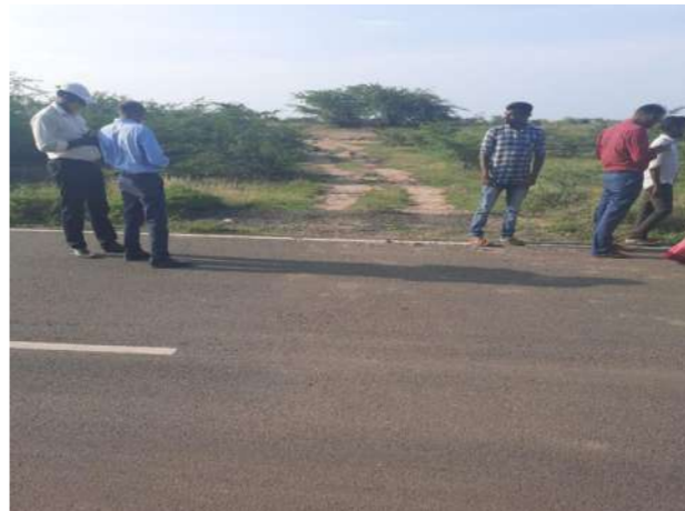
Hydrological problem- Surplus course from 560 feet weir with no culvert, starting point of Peeyar river. It has no culvert, Priority is to is to construct culvert for smooth flow of river.
