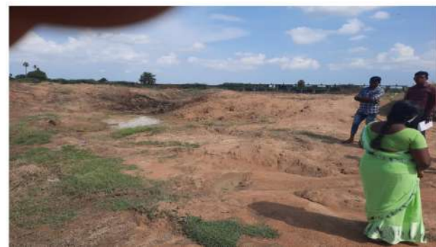
Hydrological problem- Water does not enter into the tank due to silting up of inflow point through Sarukaniar anicut to Kottakarai river. Necessary landscaping and allied works should be carried out to overcome this problem so that inflow to R.S.Mangalam tank is to be realized without any obstructions.
