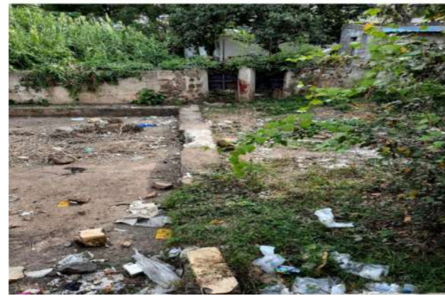
Renovation works need to be taken in Kangranandal anicut
