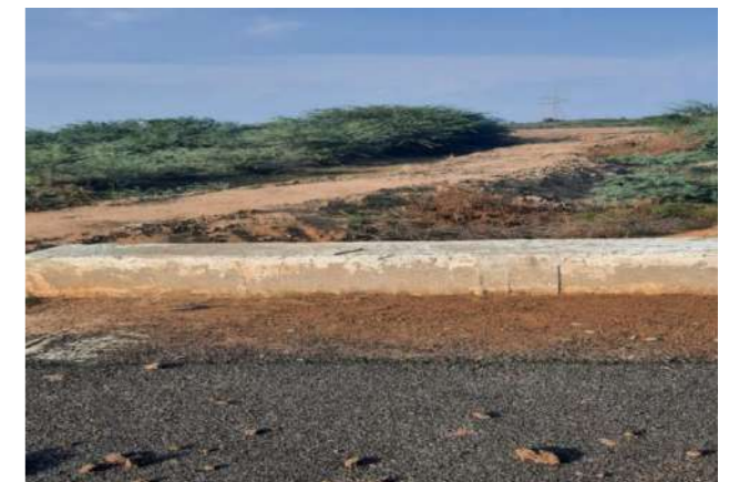
Hydrological problem- Illegal earthen bund across Peeyar river feeding Sholandur big tank which obstructing the natural flow. Rectification measures needs to be taken.
