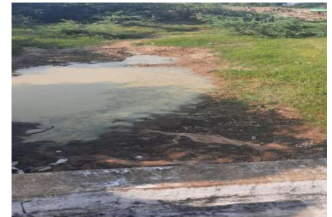
Hydrological problem - Inflow point of Vaigai River water to R S Mangalam- no dependable supply as there are lot of encroachment which needs to be removed and the entire system need to be removed.
